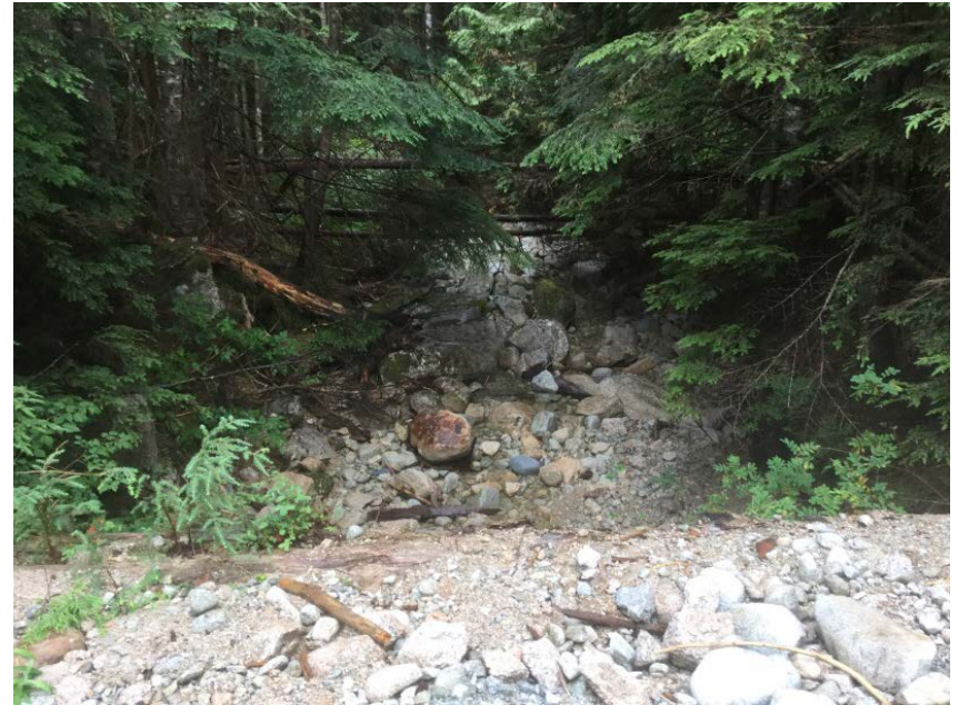
Looking downstream from deck
